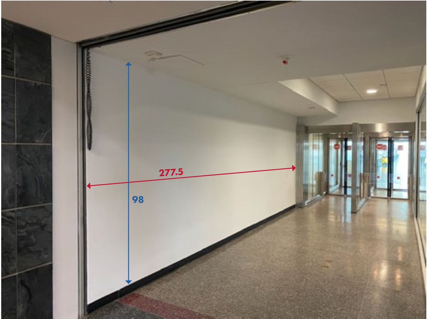
Concourse A Exit Lane Wall
